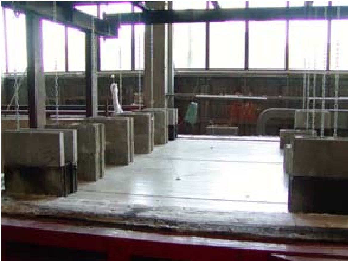
Figure 4.54: Suspended ceiling and weighted hangers on fire resistance furnace.
